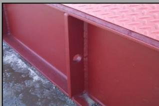
There are (3) Pulling Lugs pre-welded to each end of each section for a total of (12). These lugs are reinforced to provide safe lifting and pulling locations for easy bridge installation.
