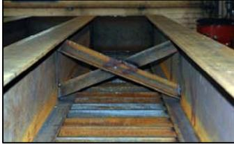
Each pad is constructed of two girders. The inside of the girders are reinforced with cross members (diaphragms). The diaphragms prevent the steel girders from twisting or bending laterally outward. Without this cross bracing, the ability of the bridge to safely carry design loads may be comprised, this is especially true of older structures that have been damaged in use or have started to corrode.
