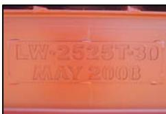
Each bridge is assigned an individual serial number for easy tracking and record keeping. Accurate records are a requirement of the OMNR Crown Land Bridge Management Guidelines – 2008.
