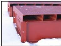
Pulling and lifting lugs are pre-welded all around the perimeter of each pad. These are extremely handy for maneuvering the bridge sections into place.
