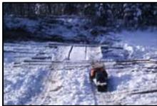
This installation consists of three pads installed side by side to provide a 12 ft. wide surface. This procedure is mostly used for skidding. This type of installation does not require any tie down spacer bars.
