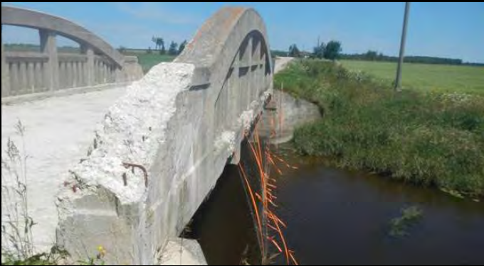
Photo 3: Downstream face of existing bridge looking southerly.
