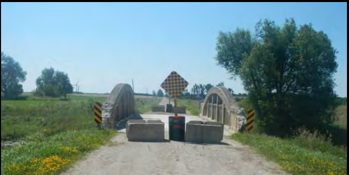
Photo 5: North approach to existing bridge with road closure barriers.
