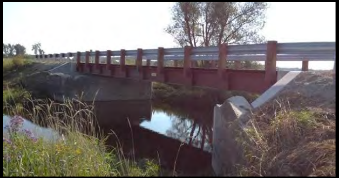
Photo 2: Upstream face of new 18.3m span Lessard Modular bridge.
