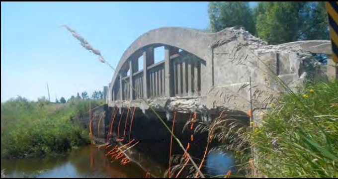
Photo 1: Upstream face of existing bridge looking southwesterly.
