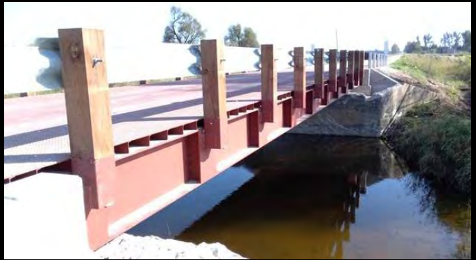
Photo 4: Downstream face of new 18.3m span Lessard Modular bridge.
