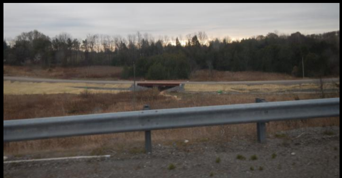
Photo 8: New 15.2m span x 6.1m wide Lessard Modular bridge from the east bound lanes of highway 401, west of off-ramp for Highway 30.
