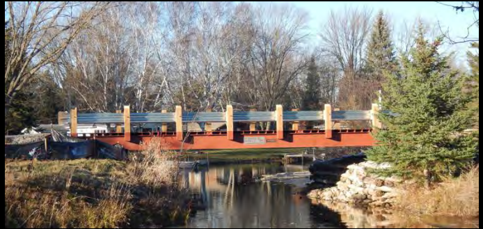
Photo 4: Downstream face of new 15.2m span Lessard Modular bridge.
