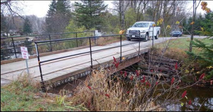
Photo 1: Downstream face of existing bridge looking NE.
