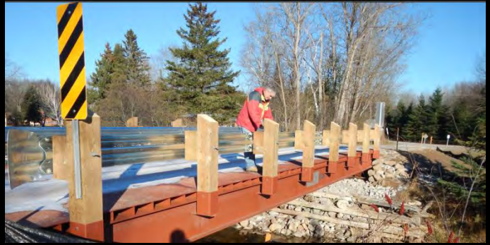
Photo 2: Downstream face of new 15.2m span Lessard Modular bridge.
