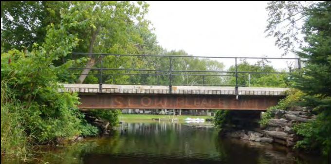
Photo 3: Downstream face of existing bridge looking N.
