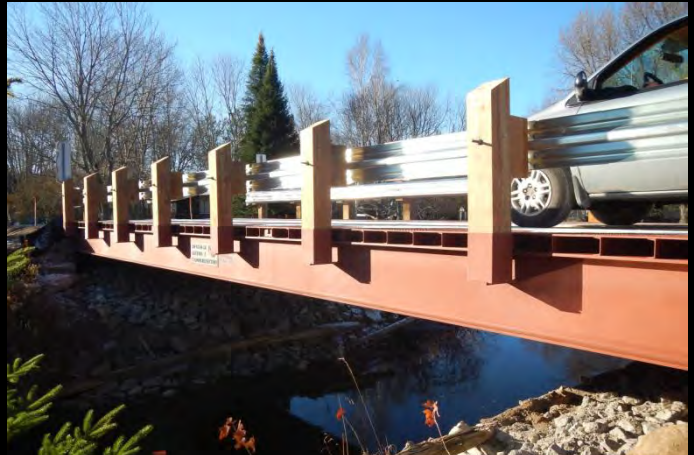
Photo 8: Close-up downstream face of new 15.2m Lessard Modular bridge - looking NE.
